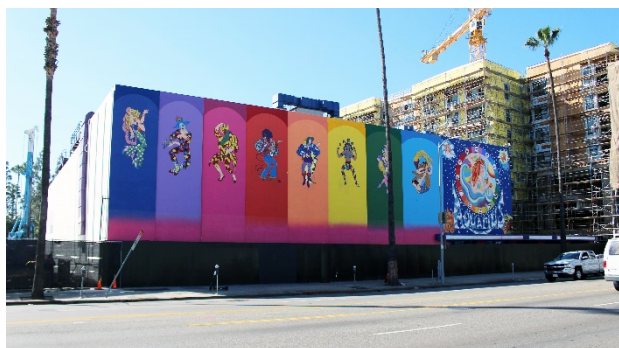
Figure 9: North and west elevations, view looking southeast, 2020 (GPA)
