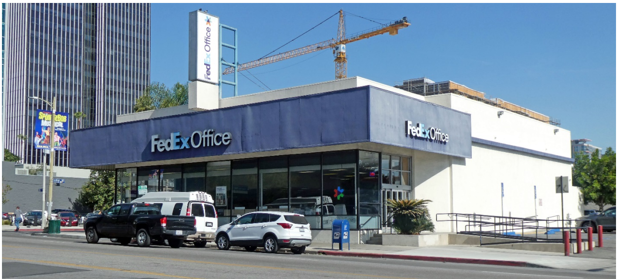
Figure 21: Primary (west) and south elevation of 1440 N. Vine Street, 2020 (GPA)
