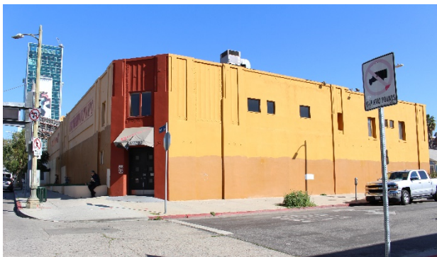
Figure 7: South and west elevations, view looking northeast, 2020 (GPA)
