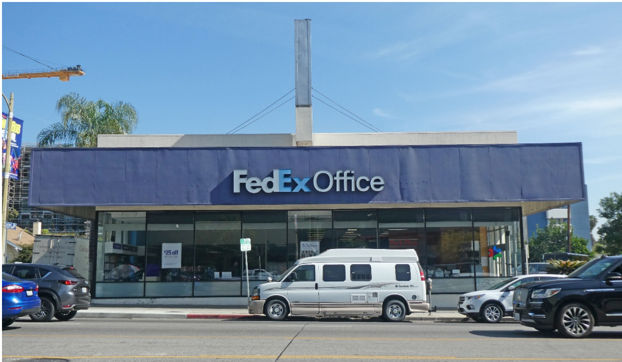
Figure 20: Primary (west) elevation of 1440 N. Vine Street, 2020 (GPA)
