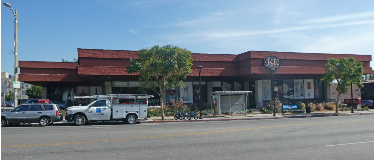
Figure 19: Primary (west) elevation of 1400 N. Vine Street, 2020 (GPA)
