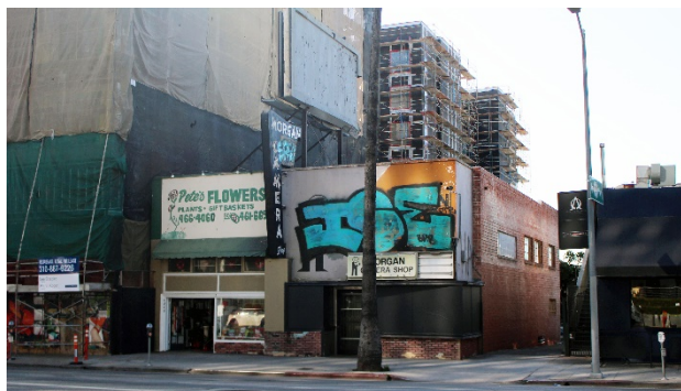
Figure 8: North and west elevations, view looking southeast, 2020 (GPA)
