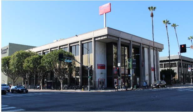
Figure 6: North and east elevations, view looking southwest, 2020 (GPA)
